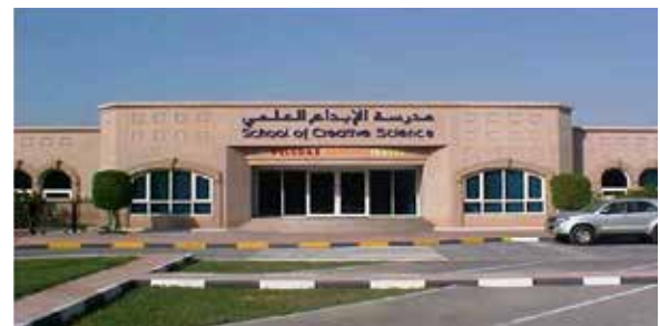
Location: Sharjah Client: Educational Investment International Contractor: Eastern International LLC
