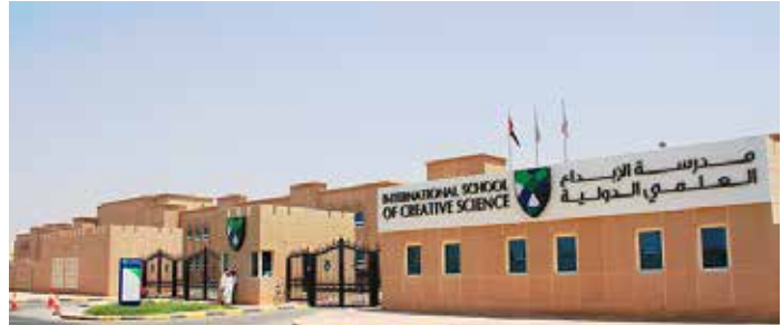
Location: Sharjah Client: Educational Investment International Contractor: Eastern International LLC
